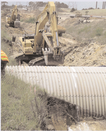
Pipeline replacement under conveyor
