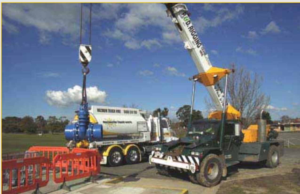
▲ Some heavy machinery had to be called in when Gippsland Water installed an additional valve to the Breed Street SPS
