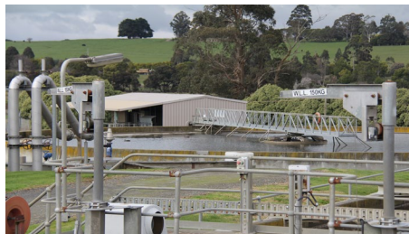
Warragul wastewater treatment plant
