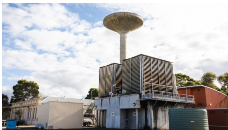
Sale water treatment plant
