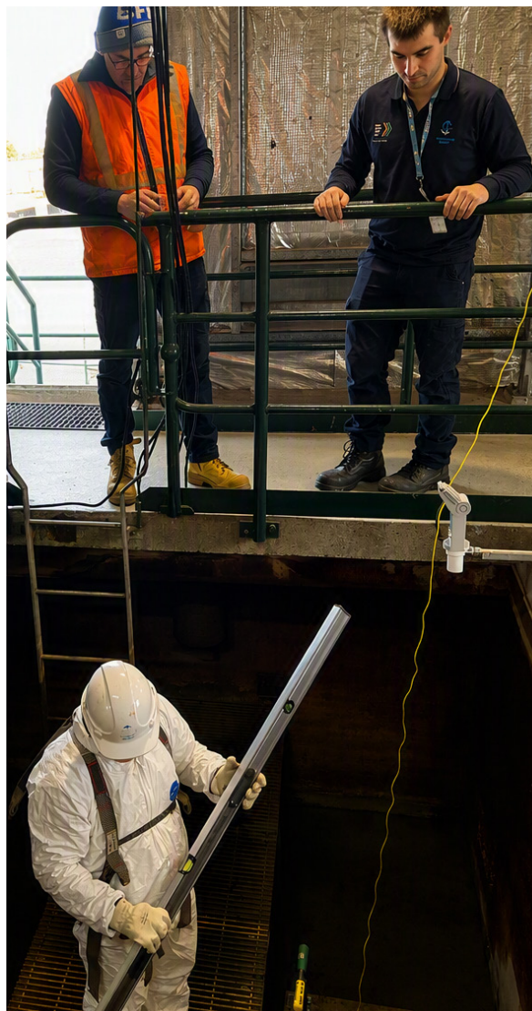
Filter inspection at Morwell water treatment plant
