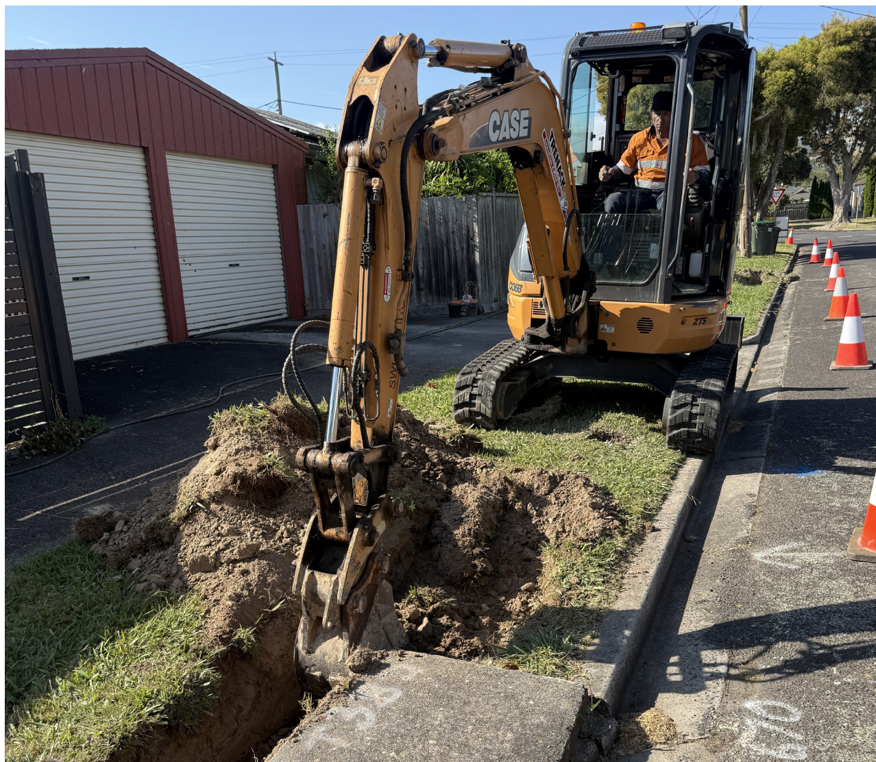
Constructing a water main
