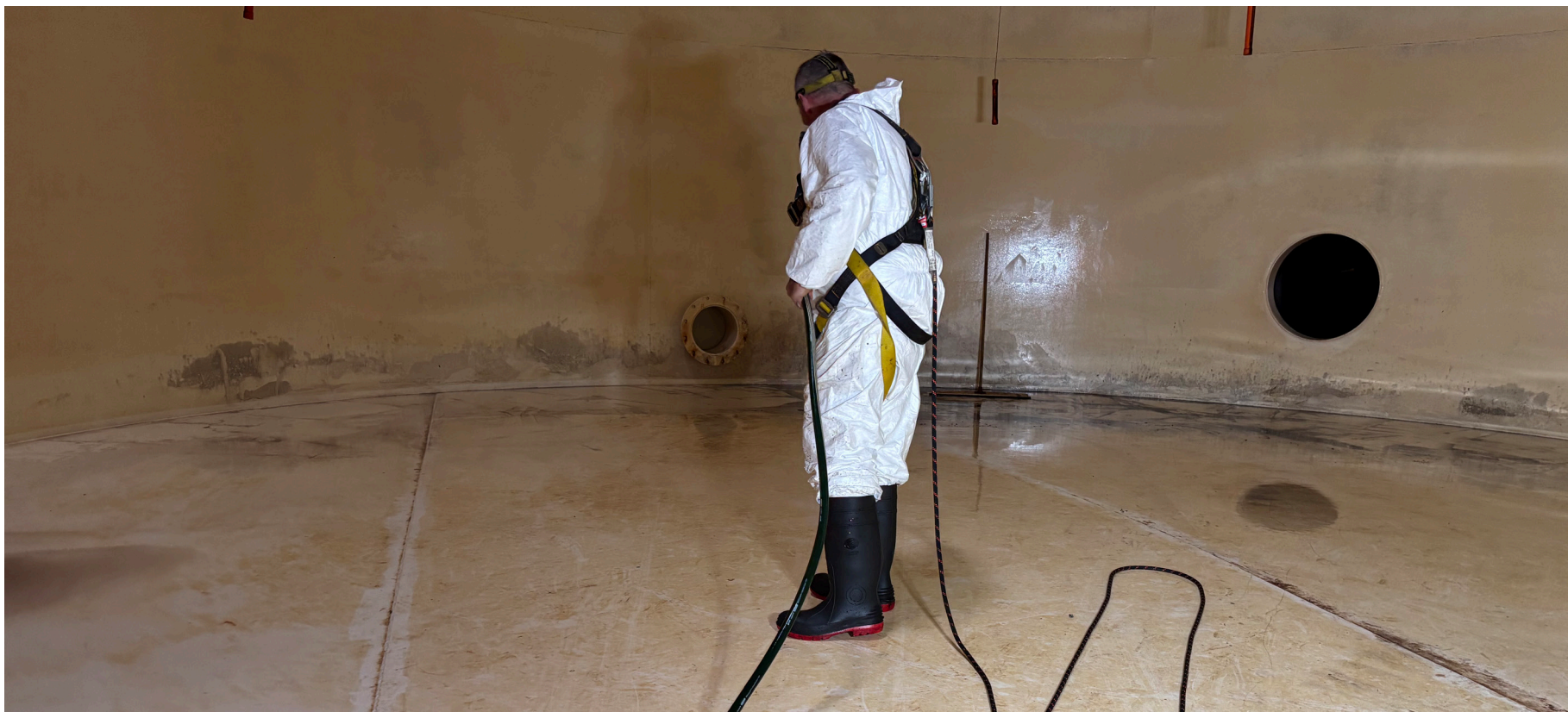
Our team cleaning the Darnum water storage tank
