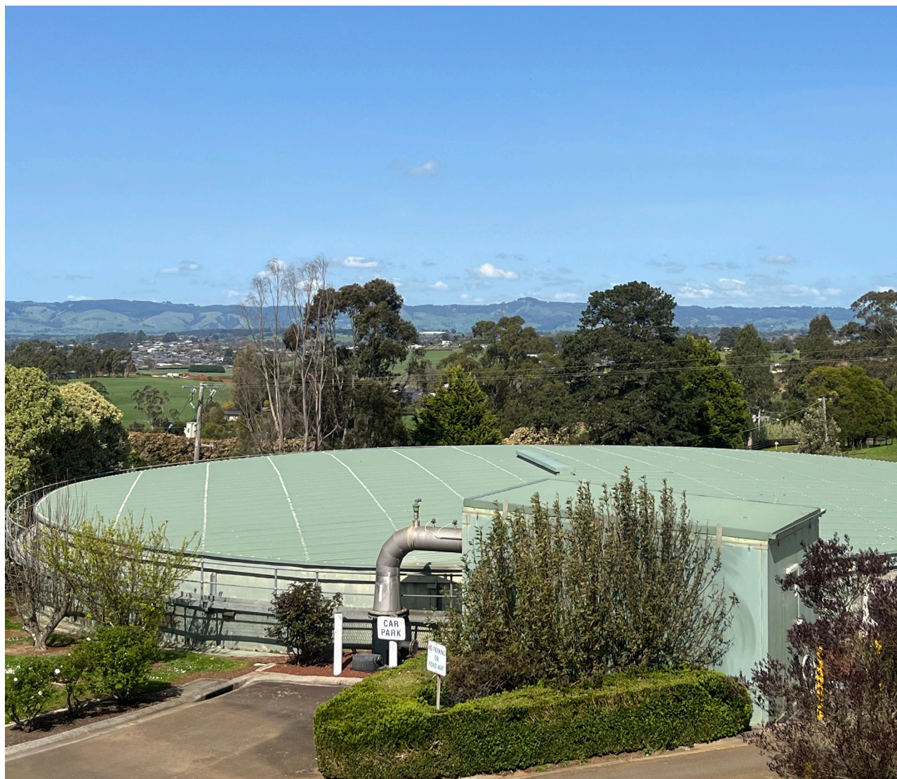
Warragul water treatment plant storage tank
