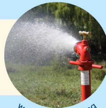
water main cleaning
